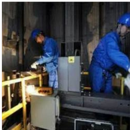
Elevator Repairing Service
