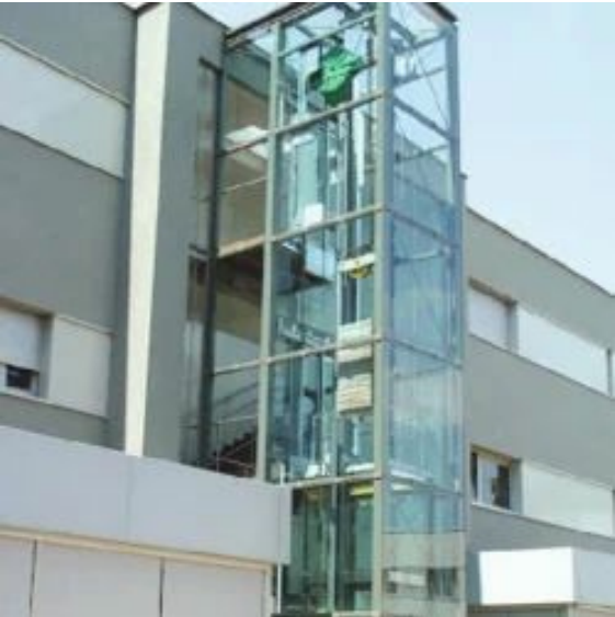
Lift Steel Structure
