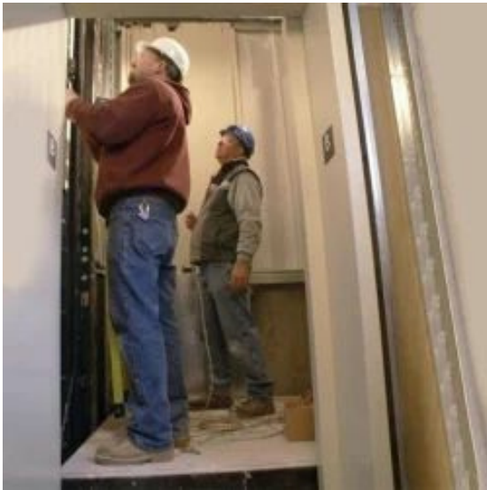
Lift Installation Services
