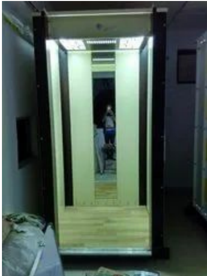
Elevator Modernization Service
